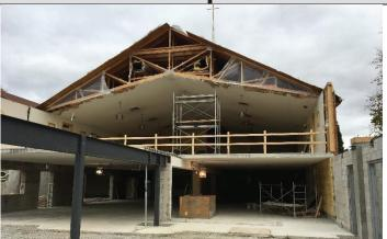
Wall removed in order to attach the original building to the newly expanded section.
