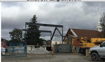
Concrete floor slabs in place for main level. Installation of metal framing has begun.
