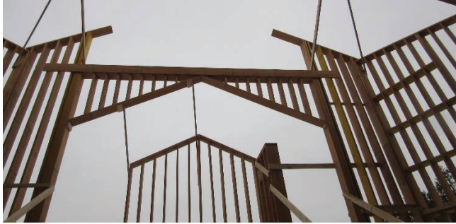
Framing around the window on the south wall
