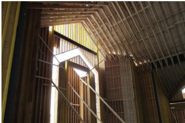
Inside and outside view of the framing for the stained glass windows
