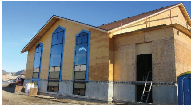
Glass windows installed
