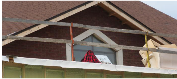
Outside walls insulated and brick work started.
