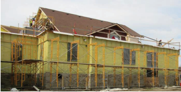
Outside walls insulated and brick work started.
